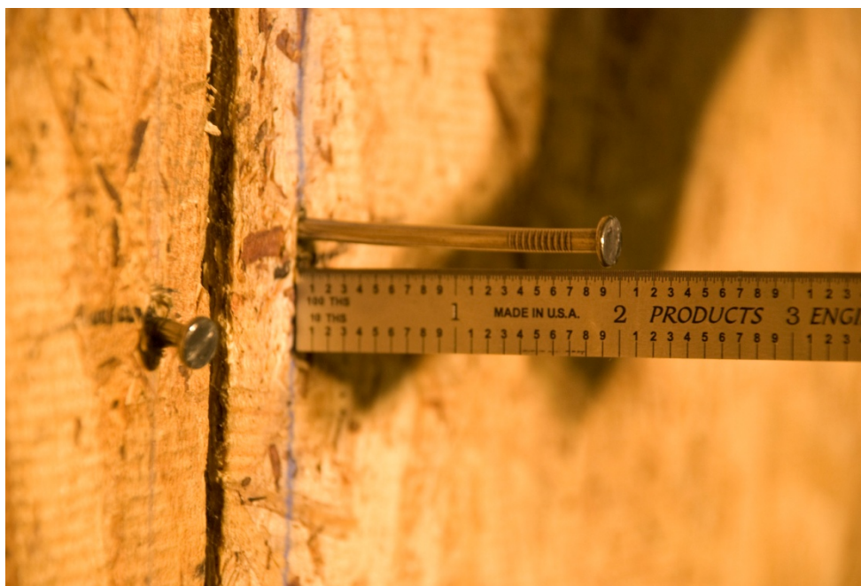
Figure 4.58: Nail pull-out along spline of Specimen A1-2C after Fatigue 3
