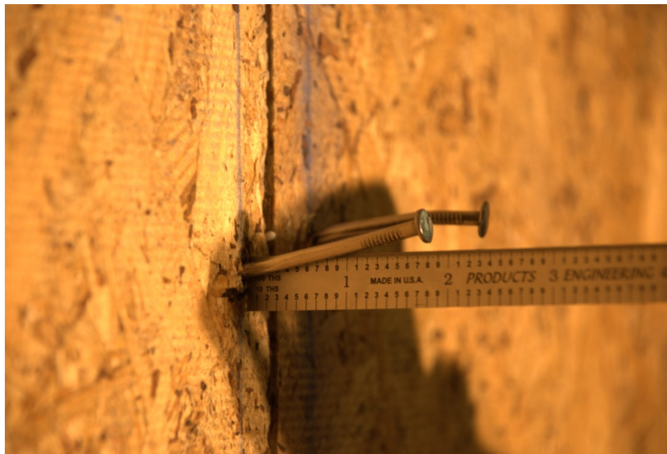
Figure 4.81: Nail pull-out along spline of Specimen A1Internal-4C after Fatigue 3
