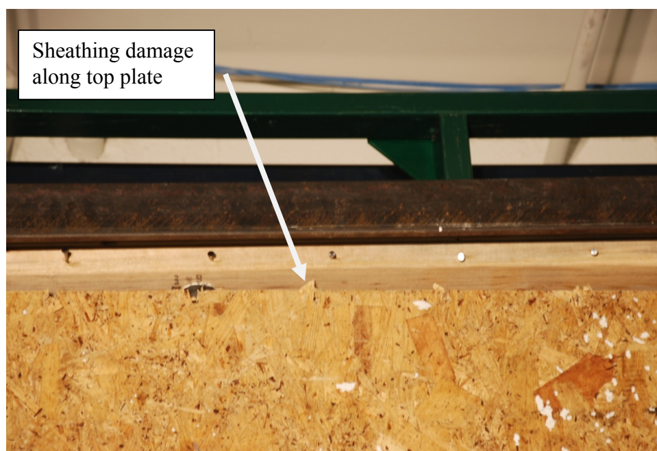
Figure 4.95: Sheathing failure along top plate of Specimen B-1C after Fatigue 1
