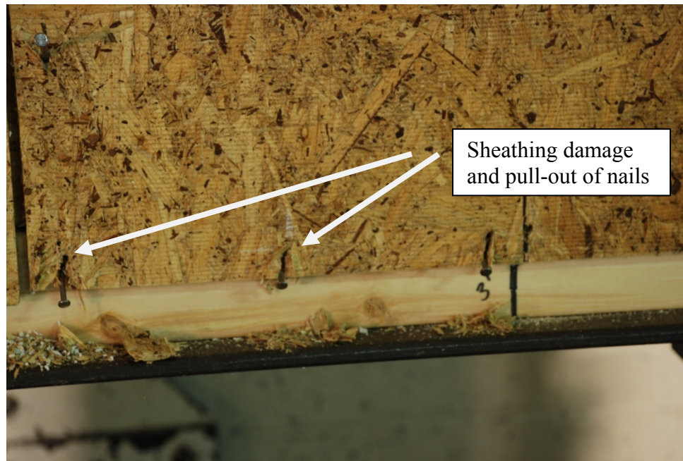
Figure 4.48: Sheathing damage along base plate of Panel 1 of Specimen A1-1C after Fatigue 3
