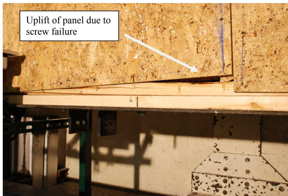
Figure 4.30: Base plate damage caused by displacement of SIP panels and failure of screws on Specimen A4-2C
