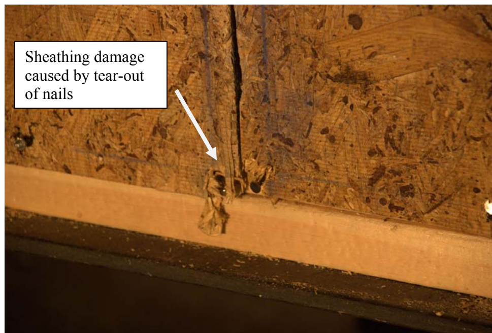
Figure 4.76: Sheathing damage at inner corner of panels along base plate after cyclic loading of Specimen A1Internal-4C
