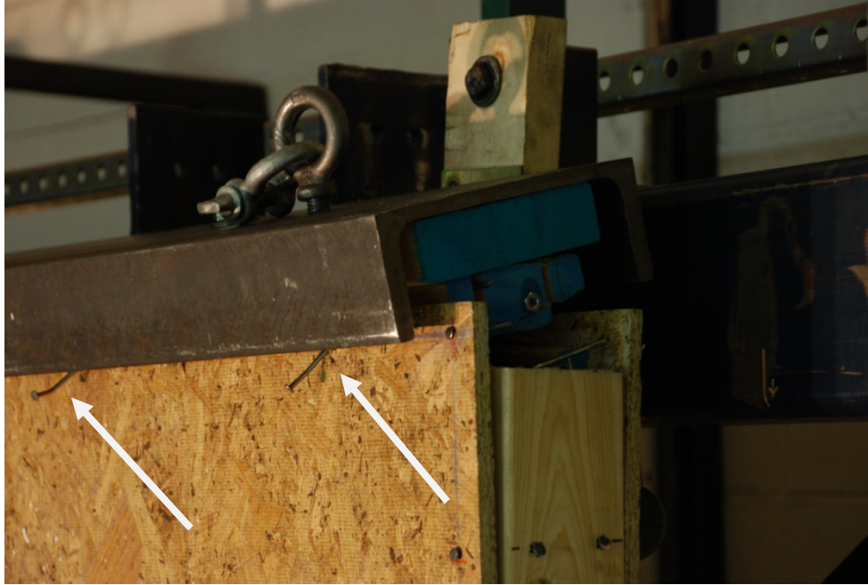
Figure 4.68: Nail pull-out along top plate (see arrows) after Fatigue 1 of Specimen A1Bearing-3C
