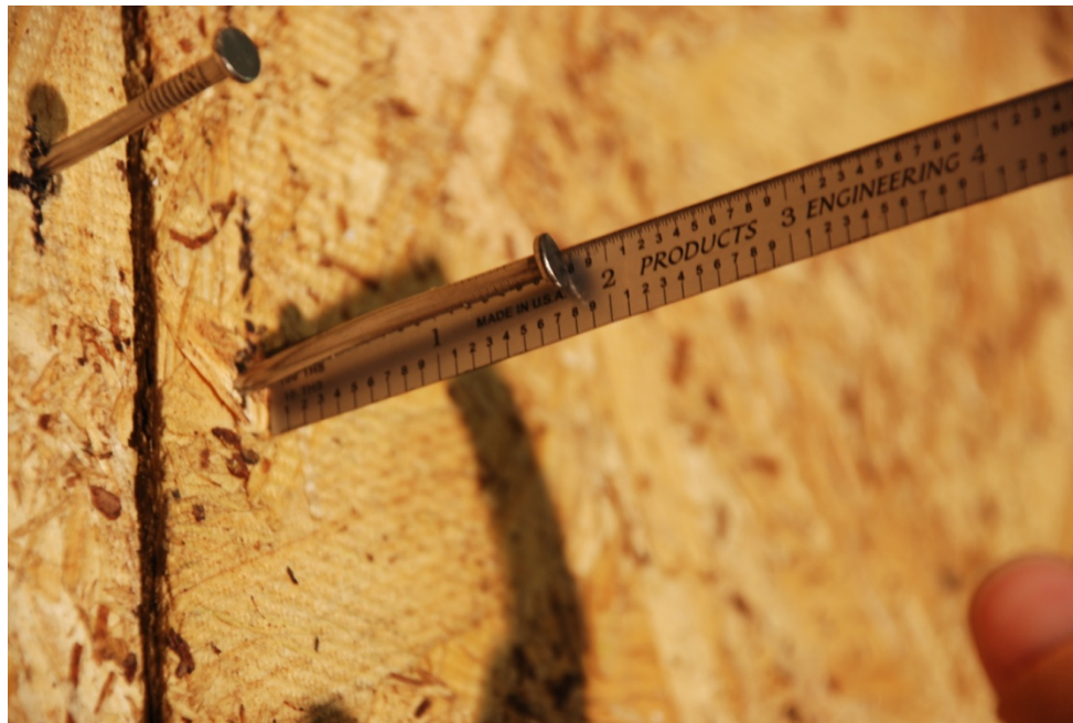
Figure 4.47: Nail pull-out along spline of Specimen A1-1C after Fatigue 1
