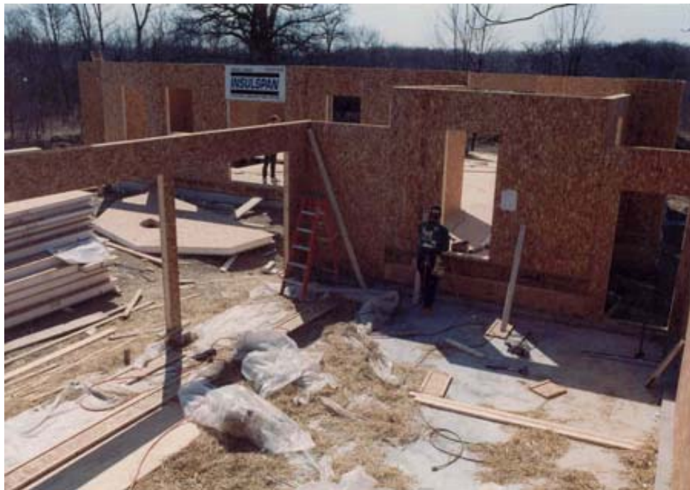
Figure 1.1: SIP home under construction (Insulspan, 2008)
