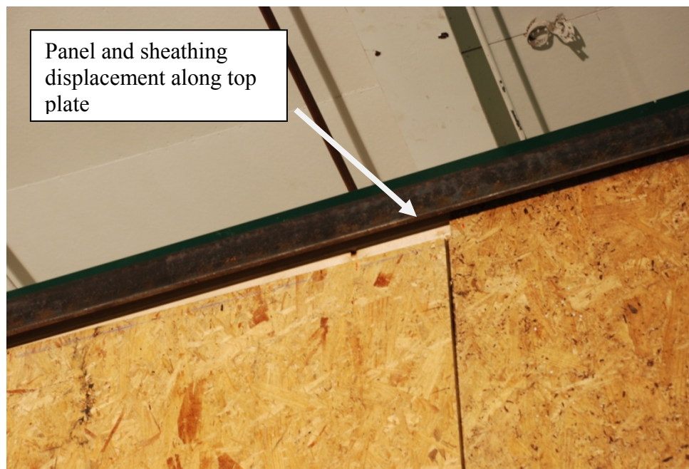
Figure 4.11: Displacement of panels along top plate after cyclic loading of Specimen A3-2C
