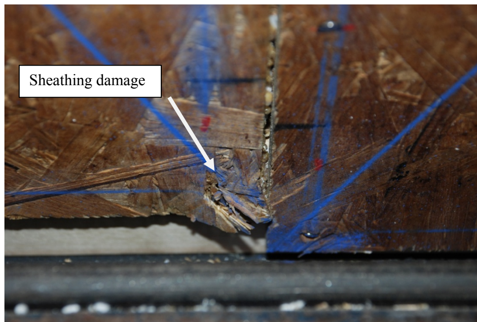
Figure 4.38: Sheathing damage at inner corner of panels along base plate of Specimen A1-1M
