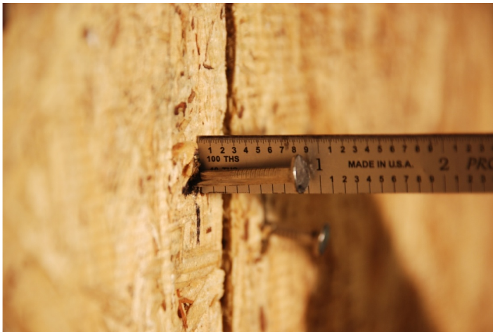
Figure 4.43: Pull-out of nail along spline after cyclic loading of Specimen A1-1C
