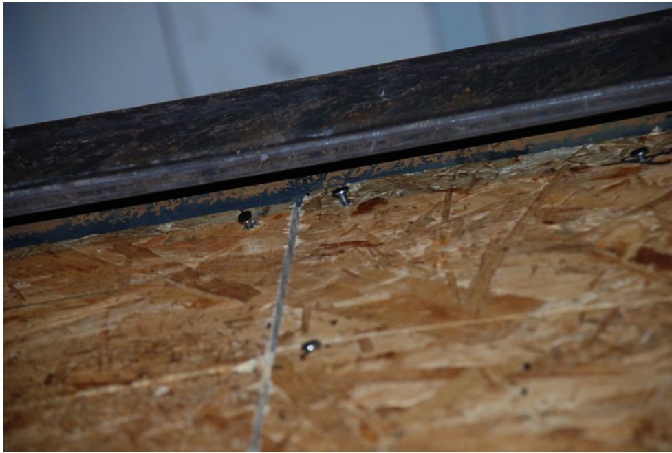
Figure 4.128: Pull-out of nails along top plate of Specimen C-3C after Fatigue 2 test
