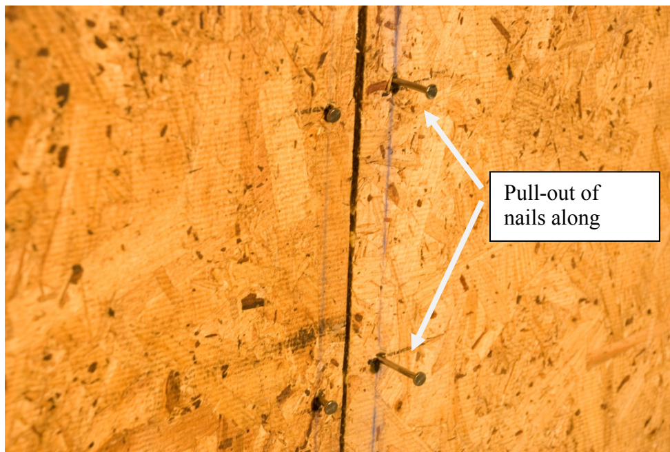
Figure 4.57: Nail pull-out along spline of Specimen A1-2C after Fatigue 1
