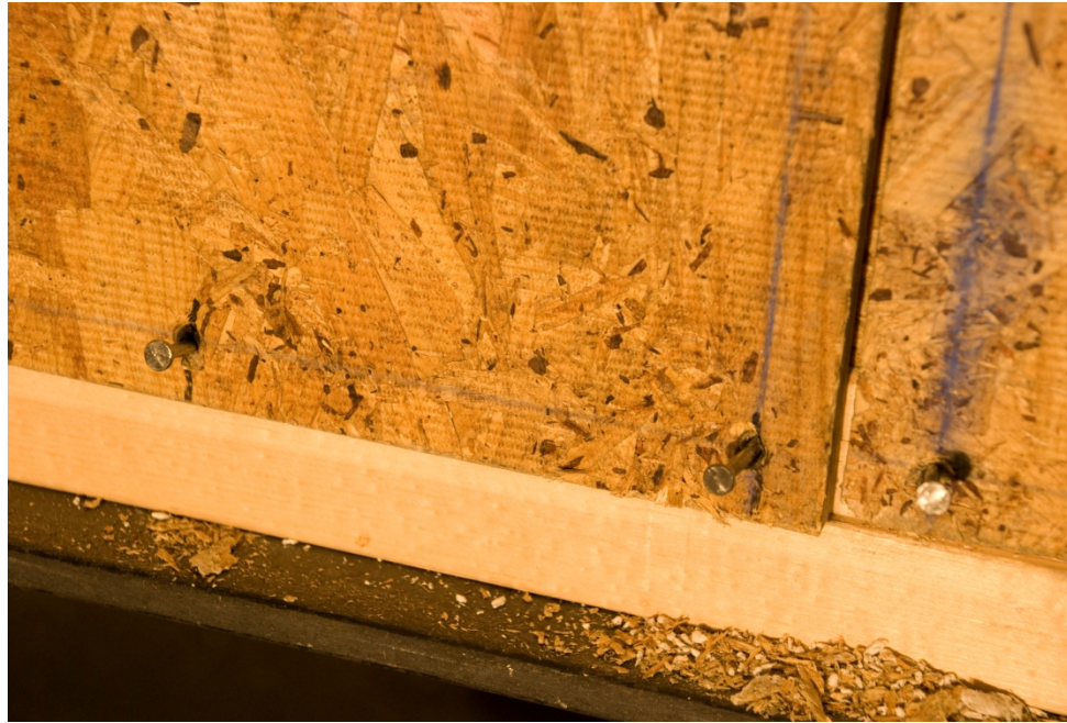
Figure 4.59: Nail pull-out along base plate of Specimen A1-2C after Fatigue 3
