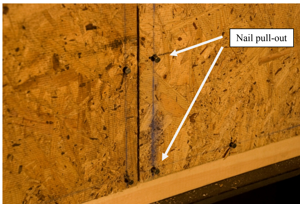
Figure 4.54: Pull-out of nails along spline and base plate caused by cyclic loading of Specimen A1-2C
