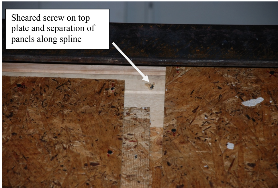
Figure 4.19: Shearing of a screw along the top plate and separation of the panel from the OSB spline of Specimen A4-1M
