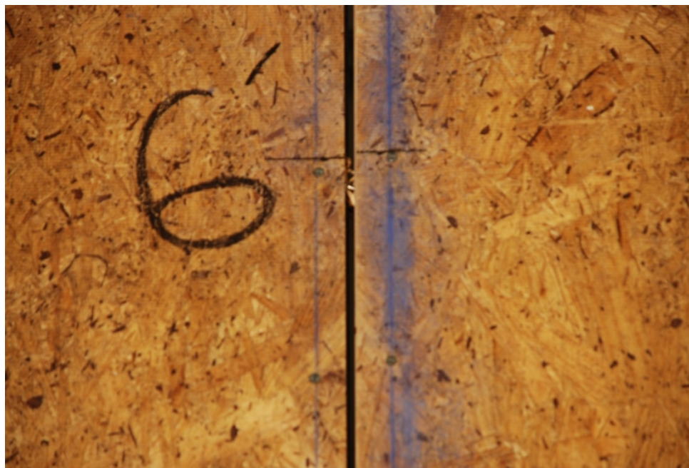
Figure 4.87: Horizontal separation of (2) 2x4 spline shown at the 6 ft high mark of Specimen B-1C after cyclic loading
