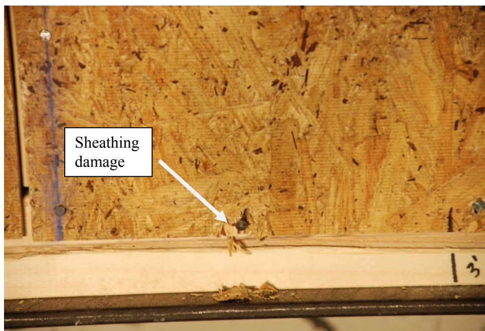
Figure 4.88: Sheathing damage along base plate after cyclic loading of Specimen B-1C
