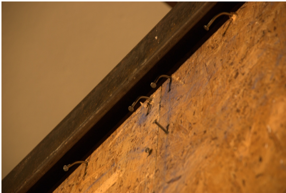
Figure 4.83: Nail pull-out along spline and top plate of Specimen A1Internal-4C after Fatigue 3
