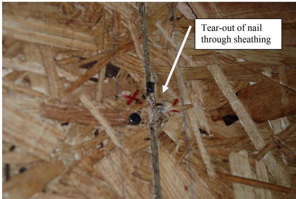
Figure 4.121: Tear-out of nail along spline of Specimen C-2C after Fatigue 2 test
